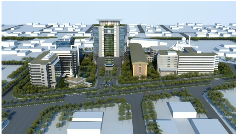
Figure 2: The Ministry of Public Works and Human Settlement Green Building Complex (EECCHI 2012)
