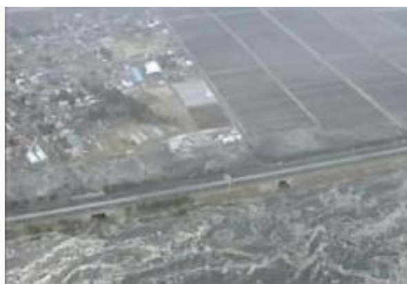
Figure 12: Disaster mitigation by the “Sendai-Tobu Road”
