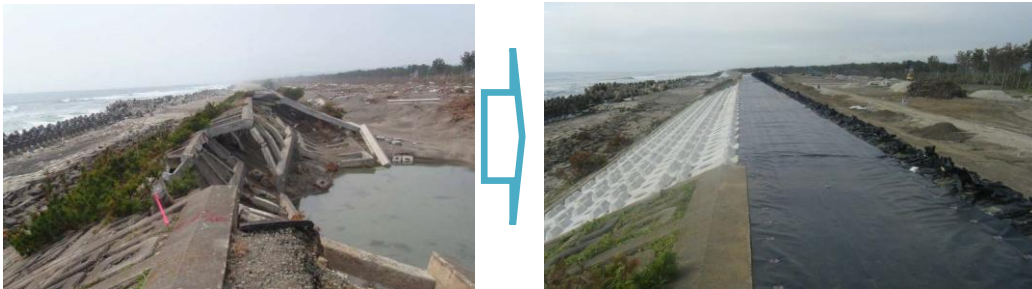
Figure 8: Emergency recovery of coast works (Iwanuma city, Miyagi Pref.)
