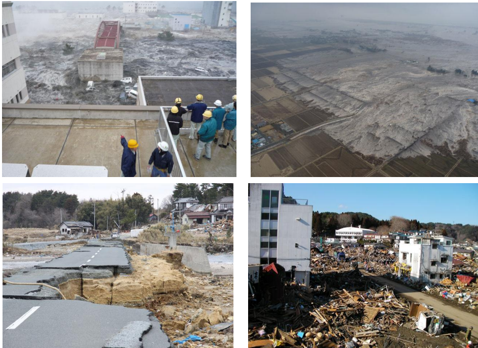
Figure 4: Damage status ②
