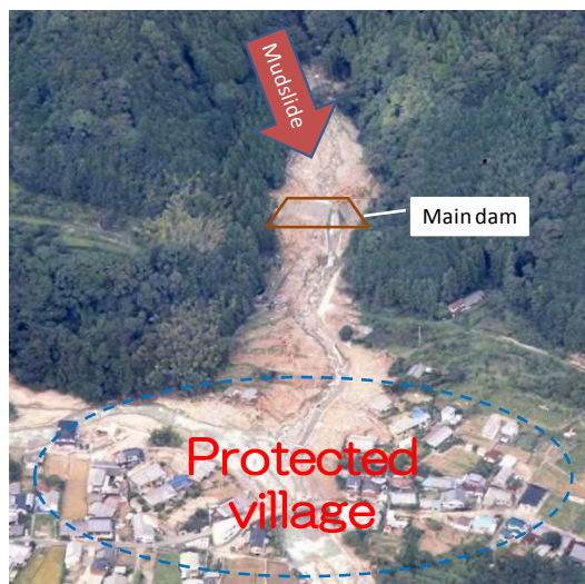
Figure 19: The effects of landslide prevention works (Wakayama prefecture)
