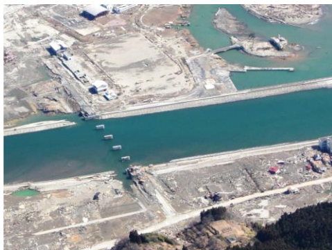
Figure 7: Emergency recovery of Bridge (Rikuzen-Takata City, Iwate Prefecture)
