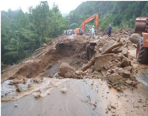
Figure 17: Emergency works on a collapsed road
