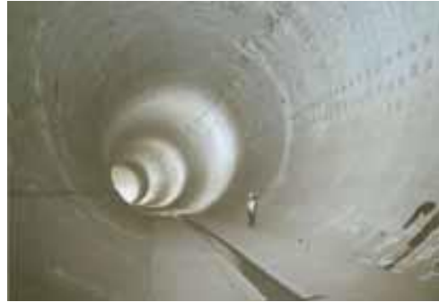
Figure 22: Underground Flood Control Reservoir
