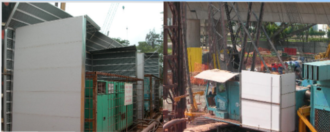
Using noise barriers to mitigate noise at source
