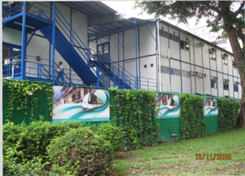
North south orientation of site office and greening of site office to reduce energy consumption.
