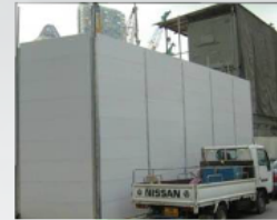
Using high hoarding as noise barrier
