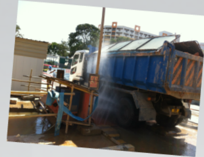
automated wheel washing bay
