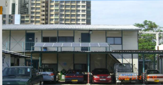
Use of solar cells for site office and powering noise meter
