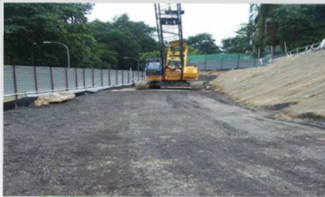
Milled waste access
