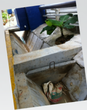
earth control measures
