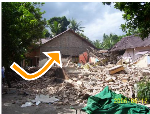
Figure 3: Two examples of the application of BARRATAGA concept by trained mandors. The two houses have stood completely with very light cracks surrounded by heavy damaged and collapsed regular houses due to the 2006 Yogyakarta-Central Java earthquake (Sarwidi et. al., 2007)
